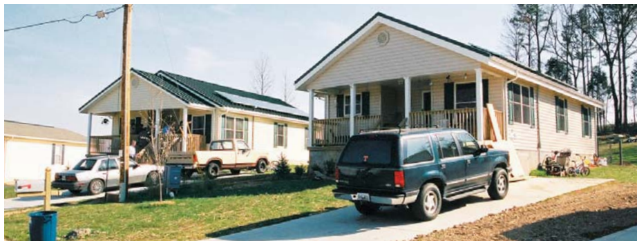
Second and third zero-energy homes constructed with EPS core panels.
