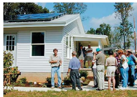
The first net-zero energy research home constructed with EPS core panels.
